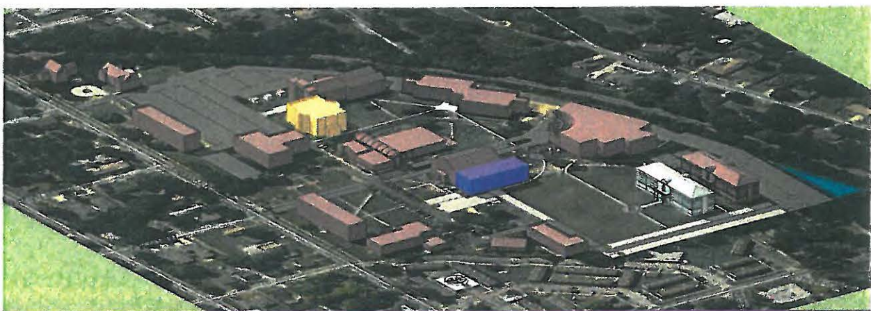
PHASE III NORTHEAST VIEW
