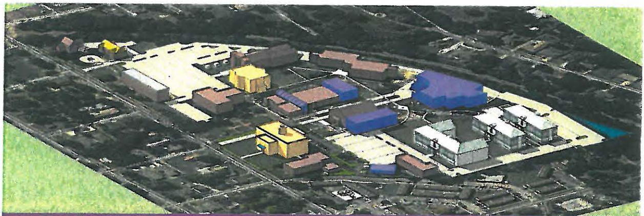
OVERALL NORTHEAST VIEW
