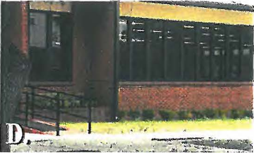
Energy efficient window upgrades throughout the campus.
